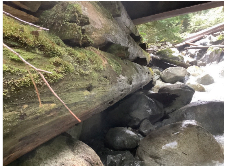
Right Bank Abutment when facing downstream
