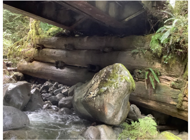
Left Bank Abutment when facing downstream
